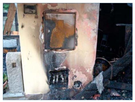
Figure 4 - Criminalistic outbreaks in the fuse box at the wooden stairs to the attic of the restaurant.
